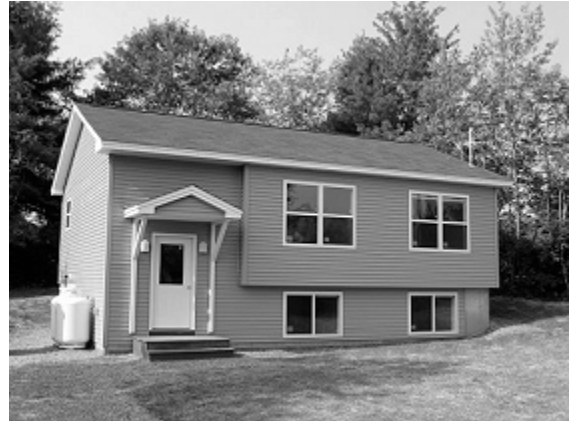
WAHFH's second home is complete.
